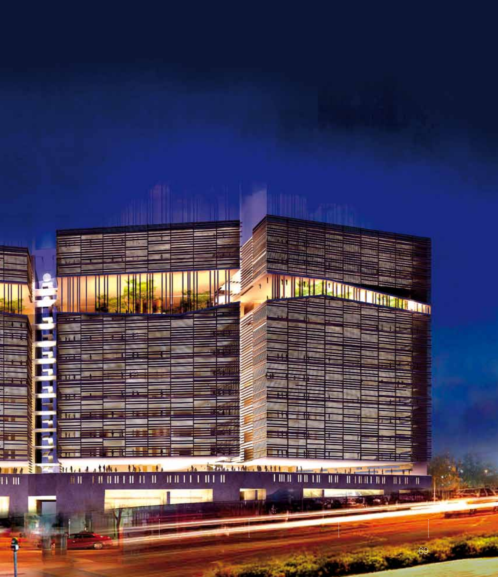
A Midnight View of the Commercial Towers at the Ersal Center
